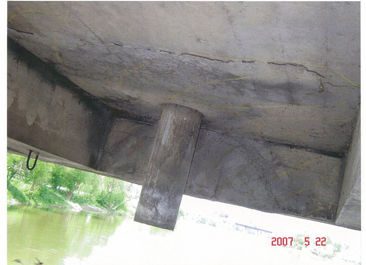
25 Typical delamination and patched areas on soffit at deck drain
