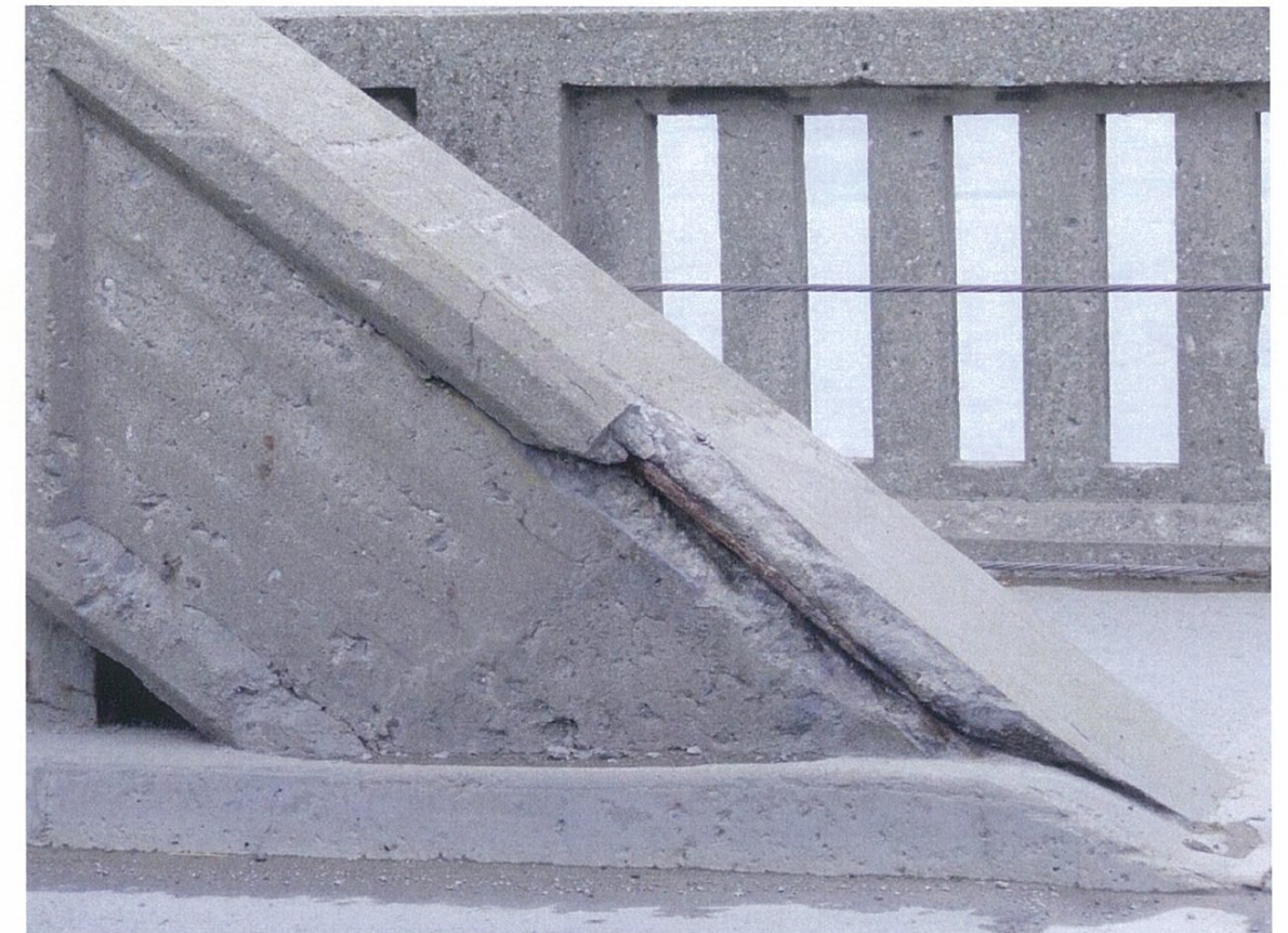
14 Cracked & Spalled south end of east arch @ Span 7
