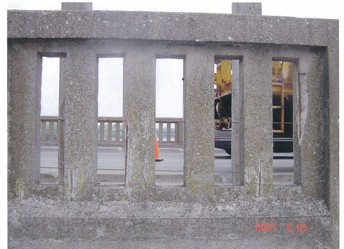
18 Delamination & Spalls on outside face of W Rail (TYP), Span 5
