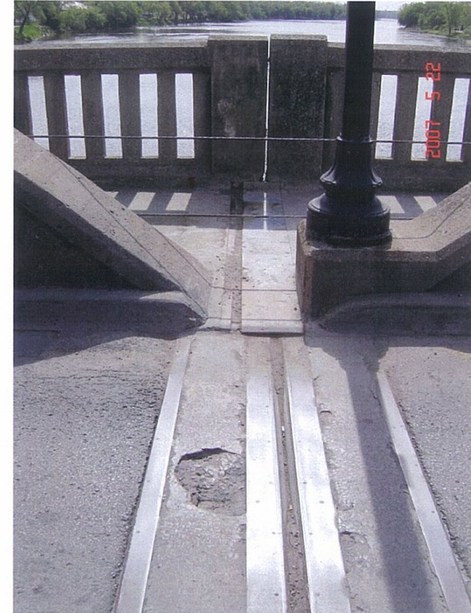
09 Local spalled on concrete end-dam (TYP)
