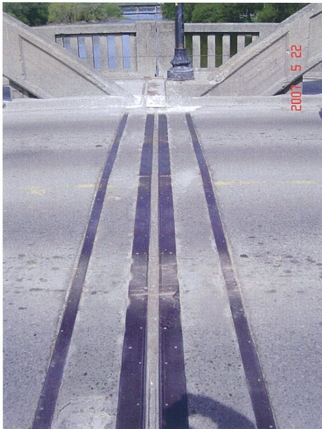
08 Typical Expansion Joint at Piers
