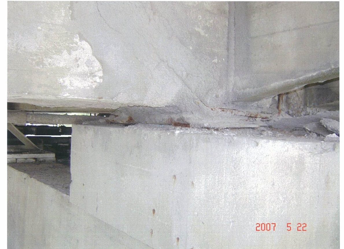
33 Exposed bent steel anchorage plate at north end of Span 8 bottom east chord, Pier 7
