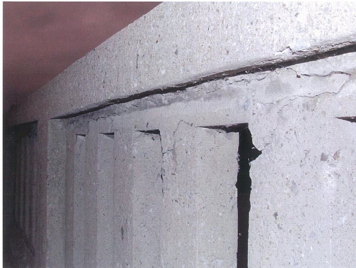
19 Lengthy horizontal crack on E rail, Span 5
