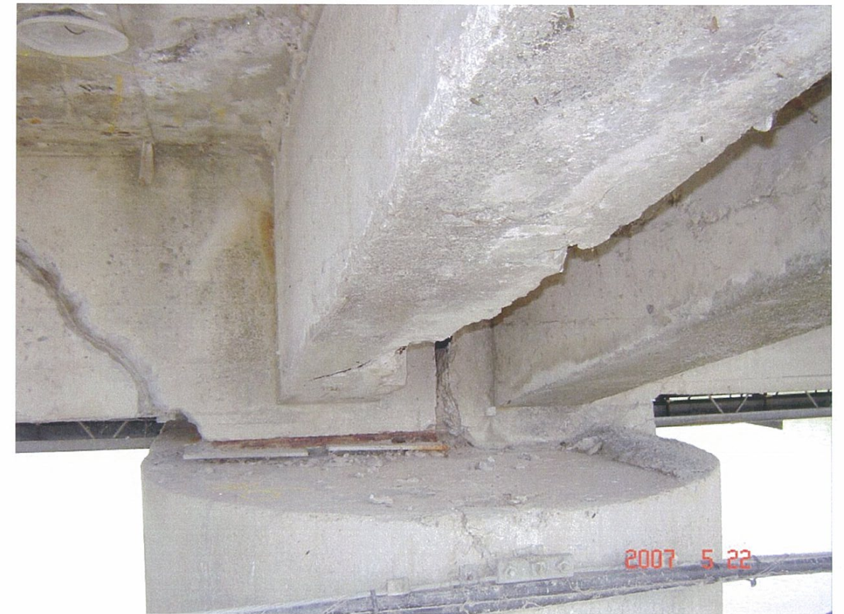
37 Typical bridge bearings, east Bearings on Pier 6 shown
