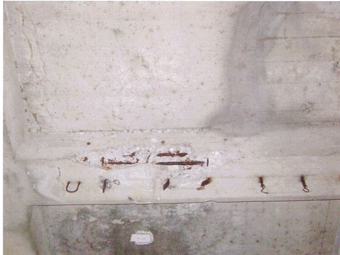
35 Typical spalled on intermediate floor beam
