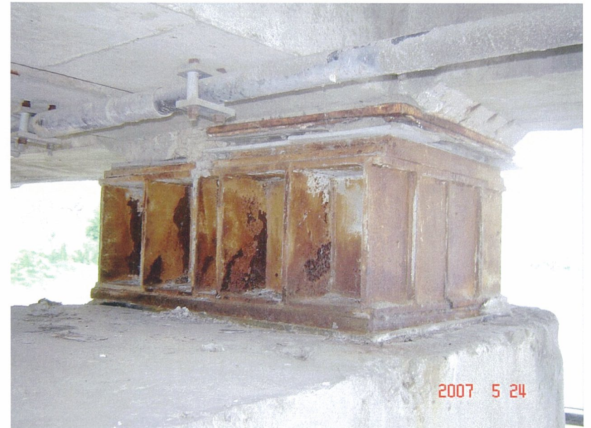
38 Steel pedestal for bearings at Pier 3 (TYP)
