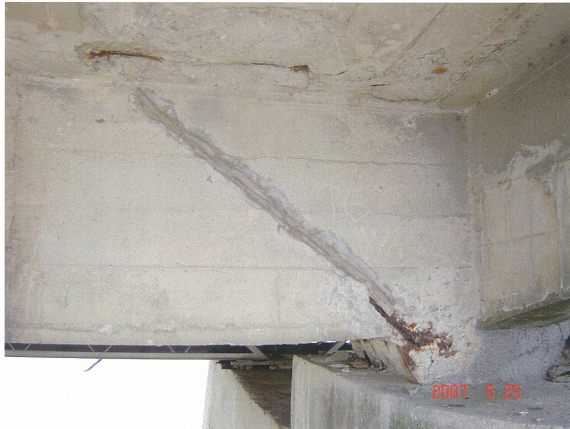
31 Sealed diagonal crack in west bottom chord west of Pier 6 (TYP)
