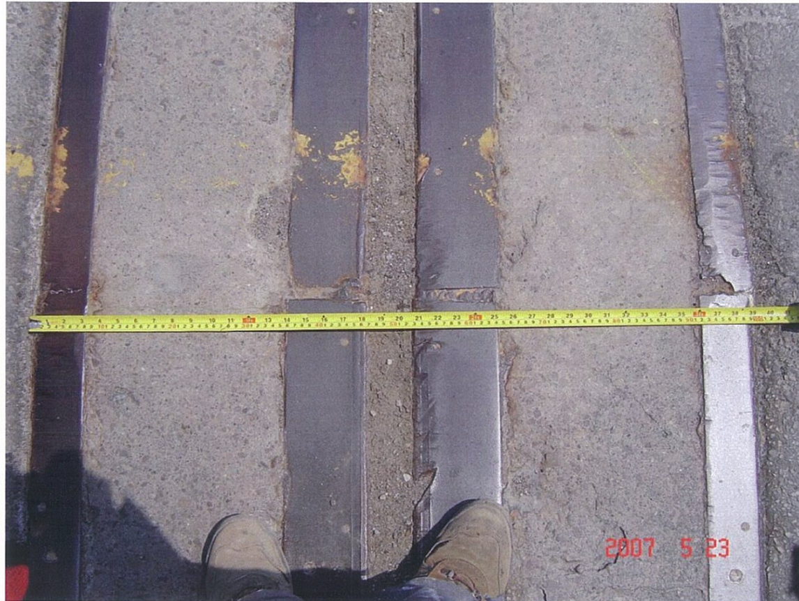
11 Damaged expansion joint armouring steel @ Pier 2 (TYP)
