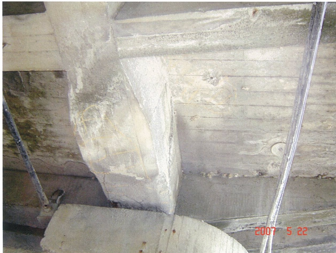
28 Typical cracked & delaminated bottom chord at end, east arch @ Pier 8 shown
