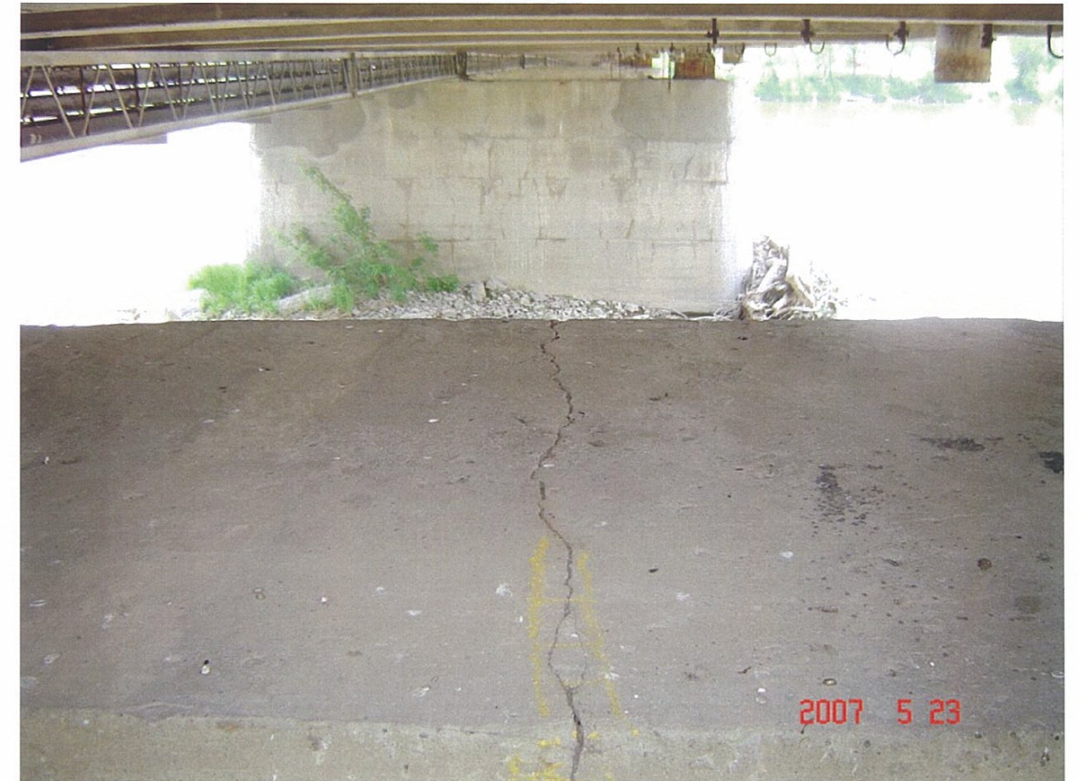
41 Wide crack across top of Pier 2
