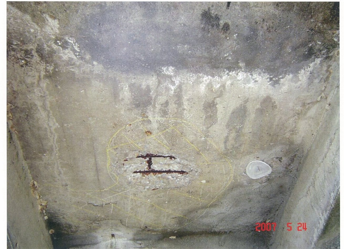
26 Typical spalled pocket on soffit
