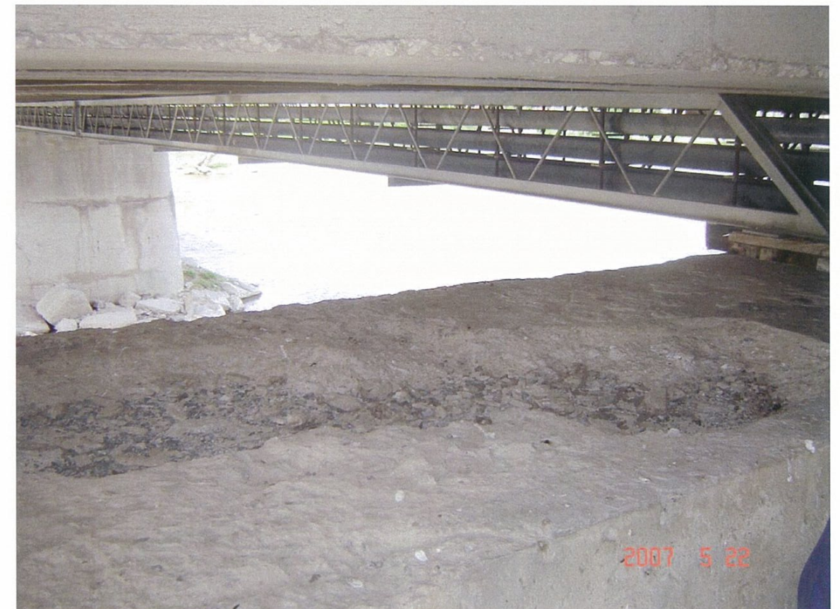
42 Local shallow spalled atop Pier 6
