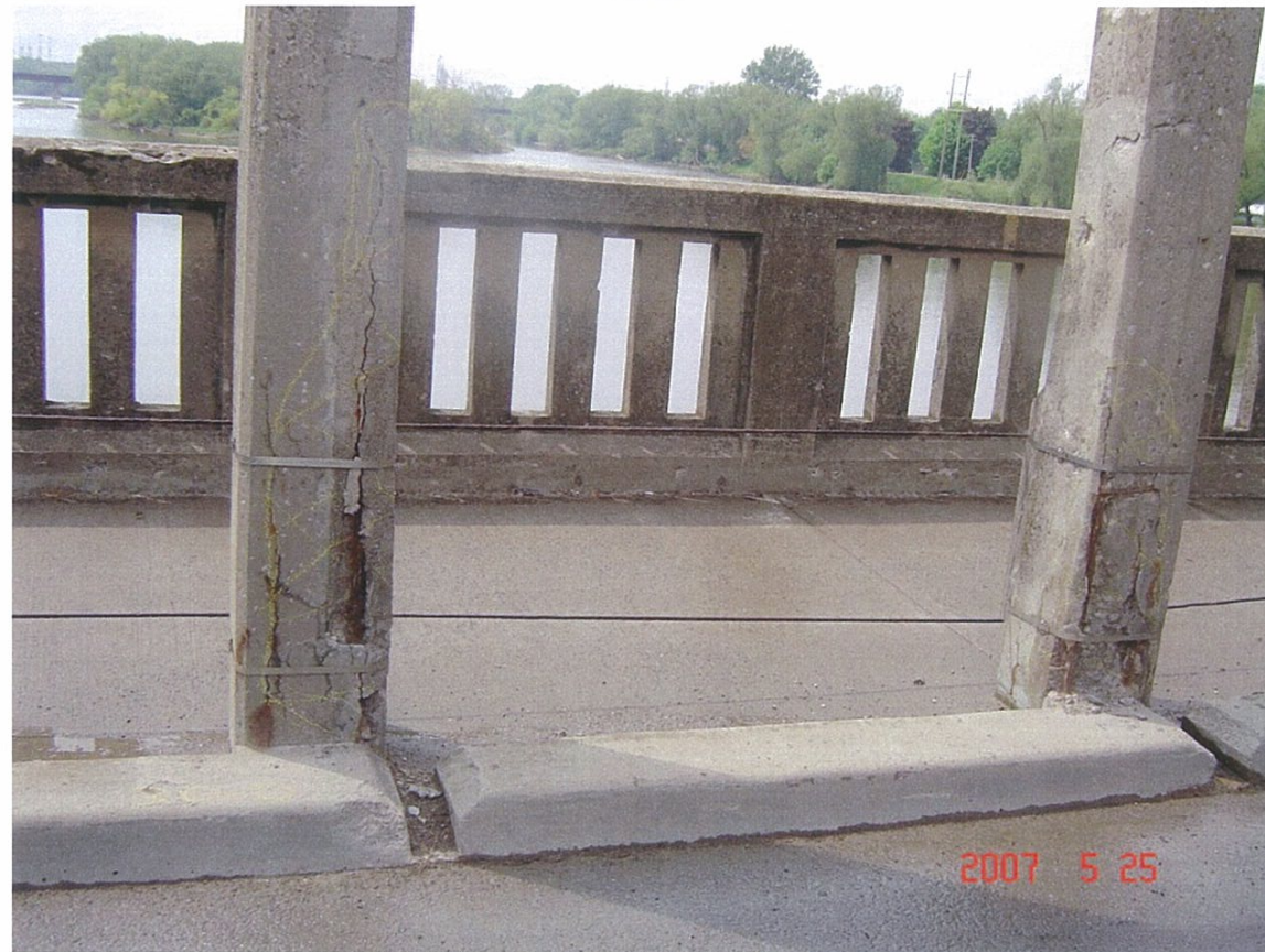
15 Typical cracks, delamination and spalls on arch hangers
