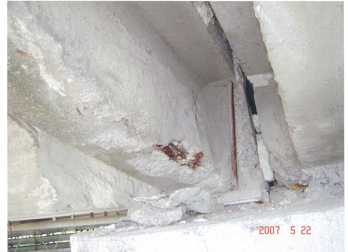
34 Spalled on floor beam under east sidewalk at Pier 7 (TYP)
