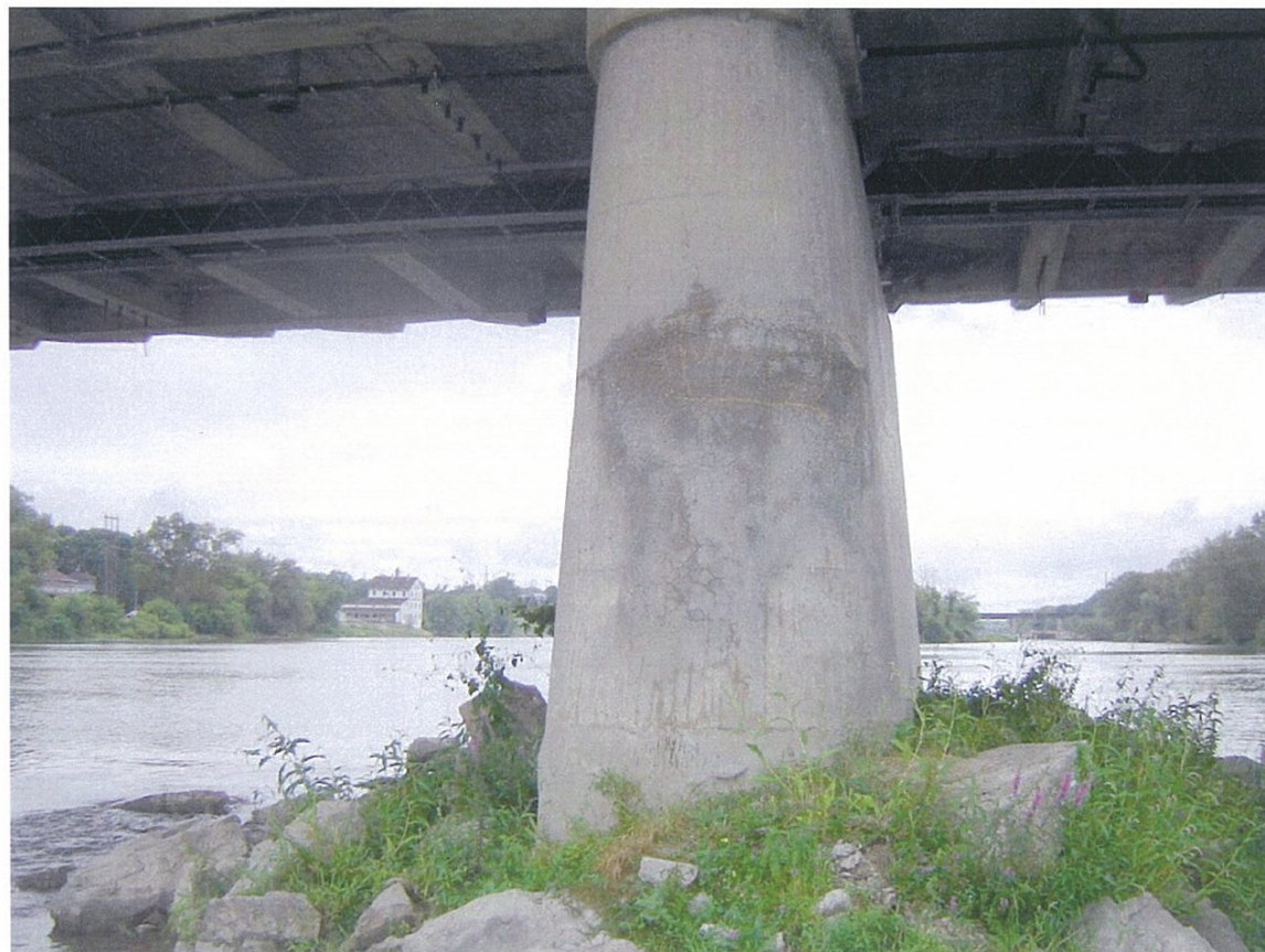
40 Localized delamination on east side of Pier 5 (TYP)
