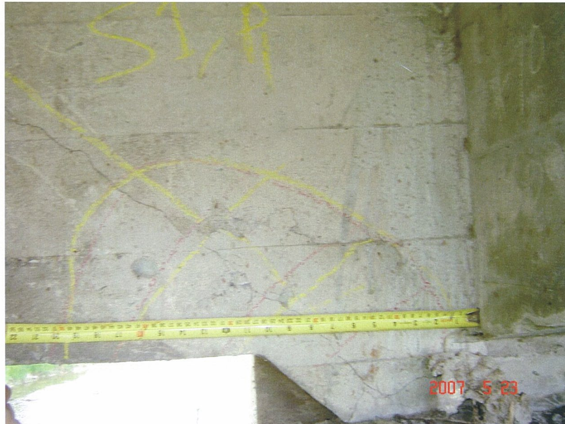
32 Diagonal crack on bottom west chord, south of Pier 1 (TYP)
