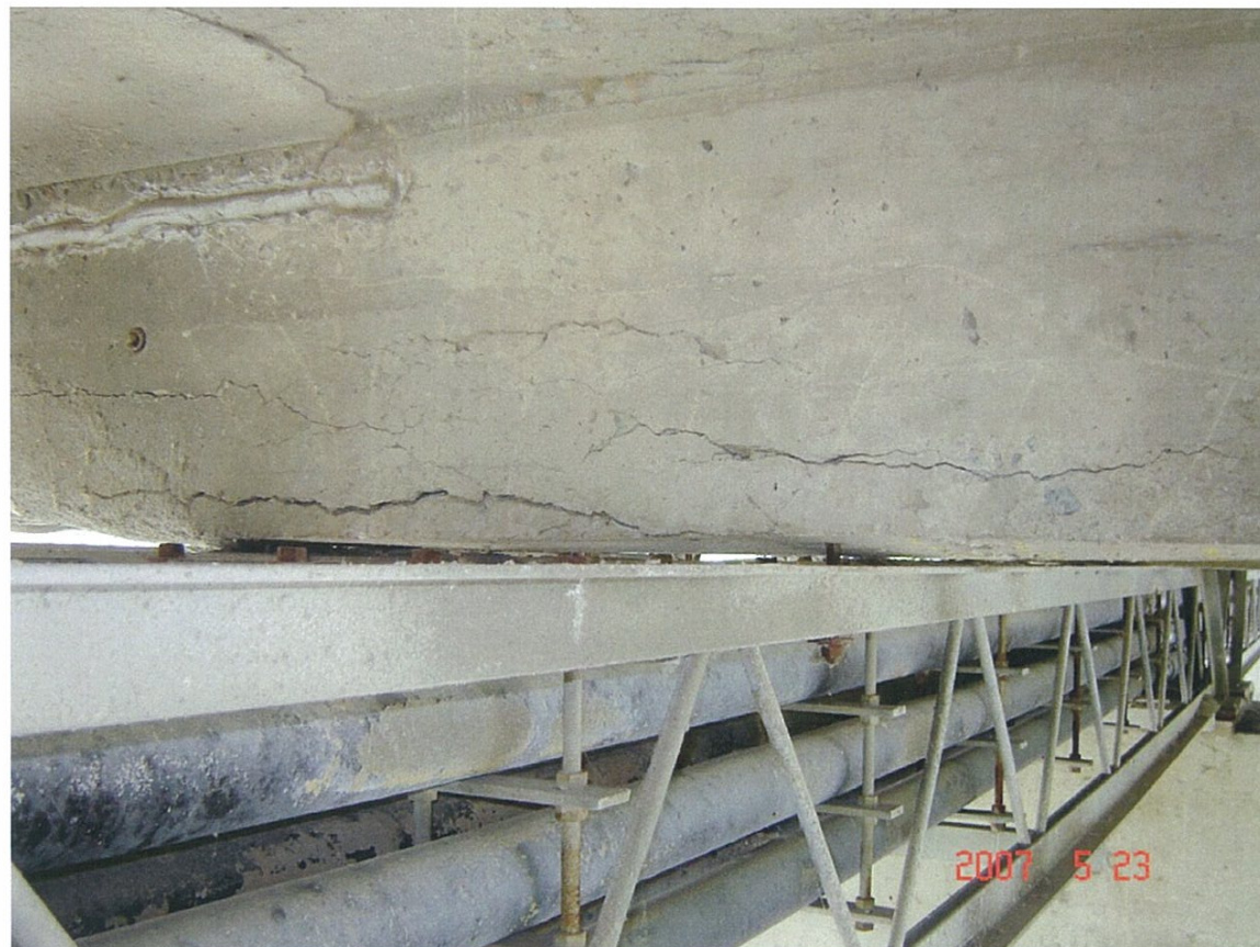
36 Cracked and delaminated interior floor beam at Span 2
