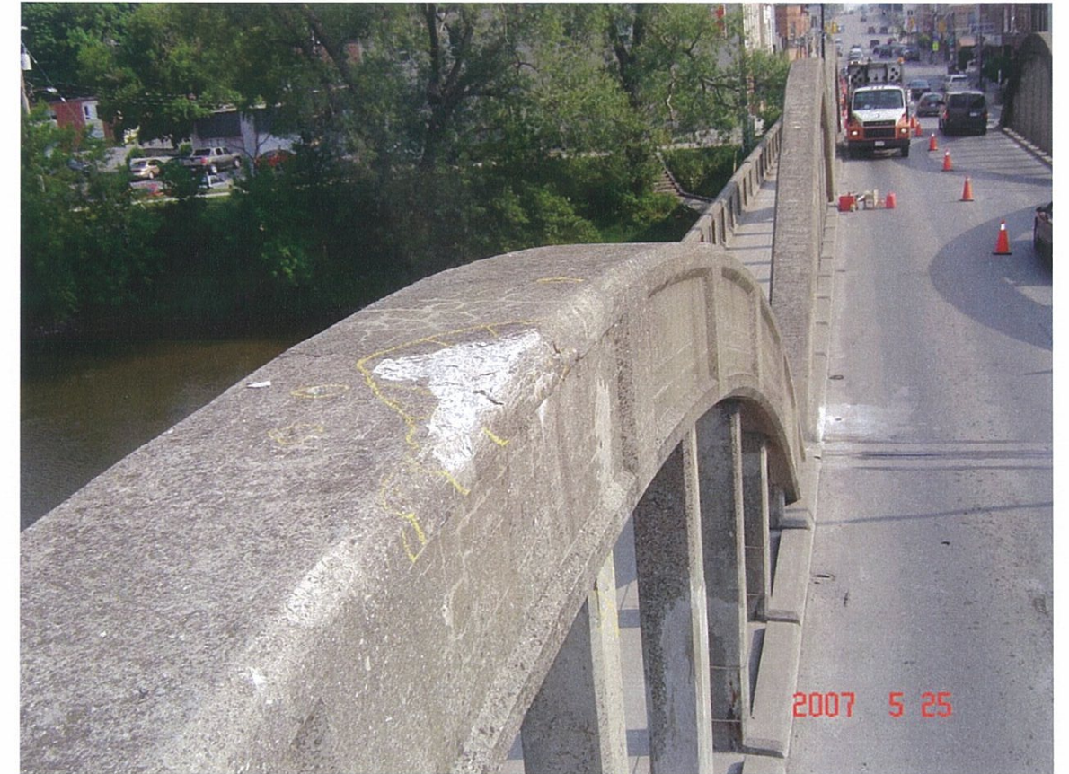
13 Minor delamination & spalled at top of W arch, Span 3
