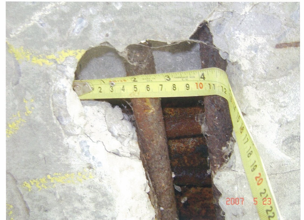
30 Exposed bars in cavity in bottom E chord, Span 2
