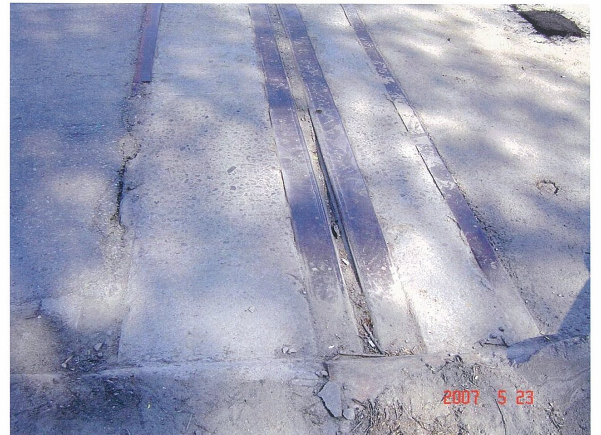
10 Missing section of armouring steel angle @ North Abutment Joint
