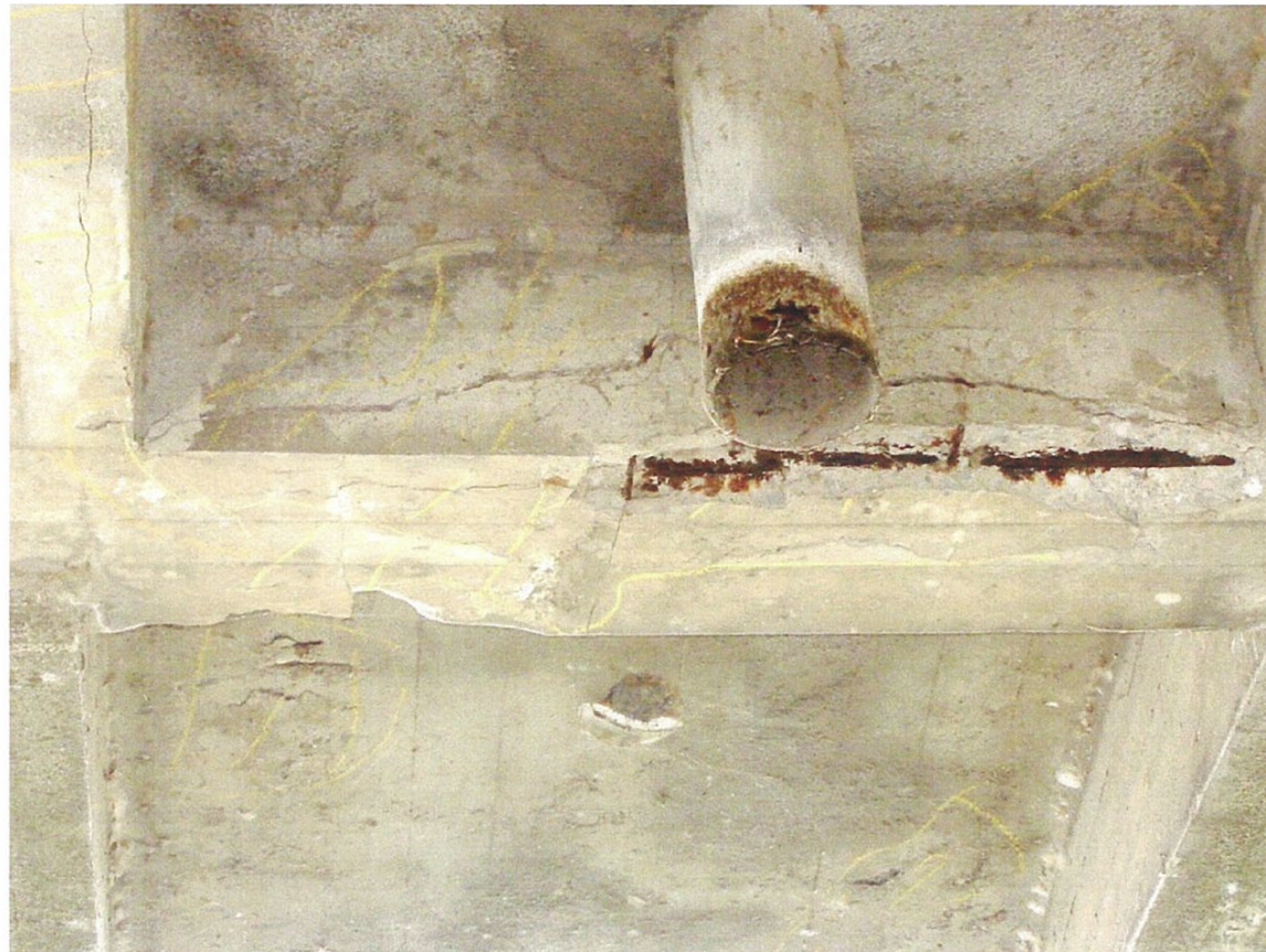
27 Cracked, Delamination and Spalled on bottom chord adjacent to a drain pipe in Span 4 (TYP)
