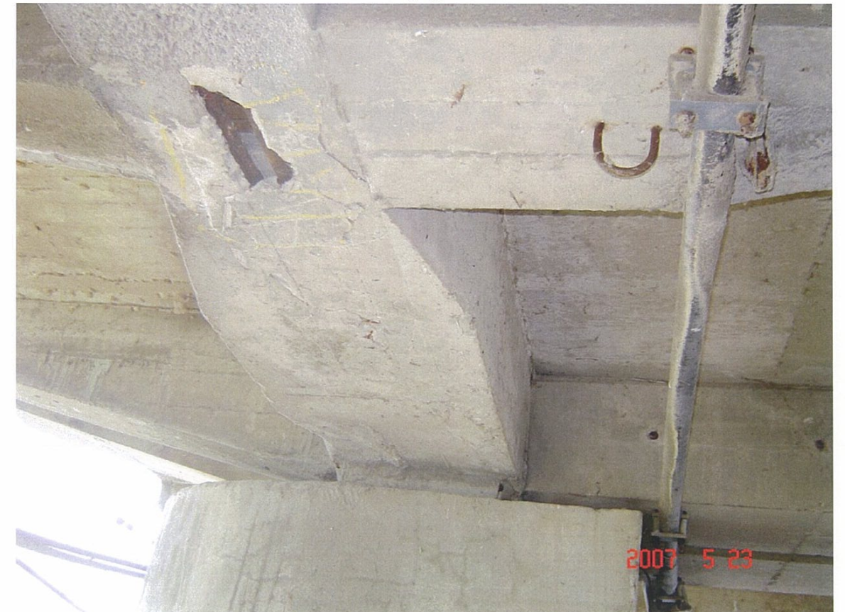
29 Large cavity in bottom E chord, Span 2
