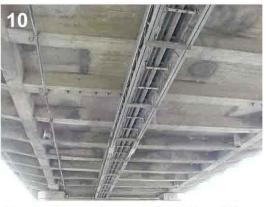
Underside of Deck in Poor Condition
