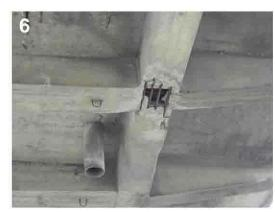
Concrete Arch Beam in Poor Condition
