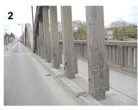
Concrete Arch Hanger in Poor Condition
