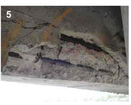
Concrete Arch Beam in Poor Condition
