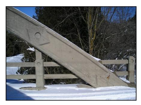
Plate 7: Decorative panels and concrete detailing on Piercey's Bridge. Source: Andreae, 2005.
