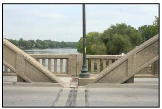
Plate 16: Truss detail with light base and expansion joints.
