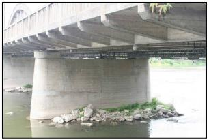
Plate 10: Pier detail with spread footing just visible below the surface.
