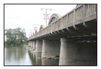
Plate 13: Cantilevered sidewalk and railing. Showing also modern bridge lighting. West side of bridge, looking north.
