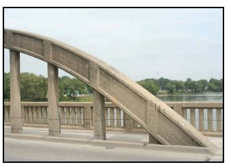
Plate 17: Concrete detailing of arch and hangers.
