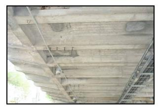
Plate 12: Bottom cord with floor beams under deck and cantilevered under sidewalk. A modern utility tray is on the right. Old utility hangers in floor beam on left.
