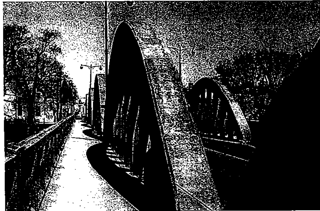
Plate 8. Sidewalk on the west side
