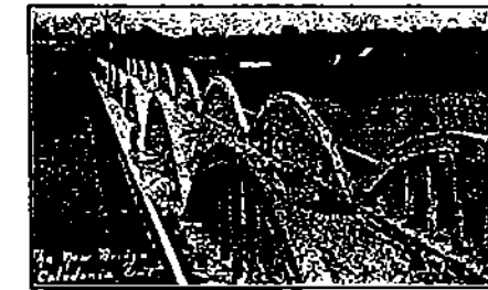
THE COMPLETED BRIDGE
