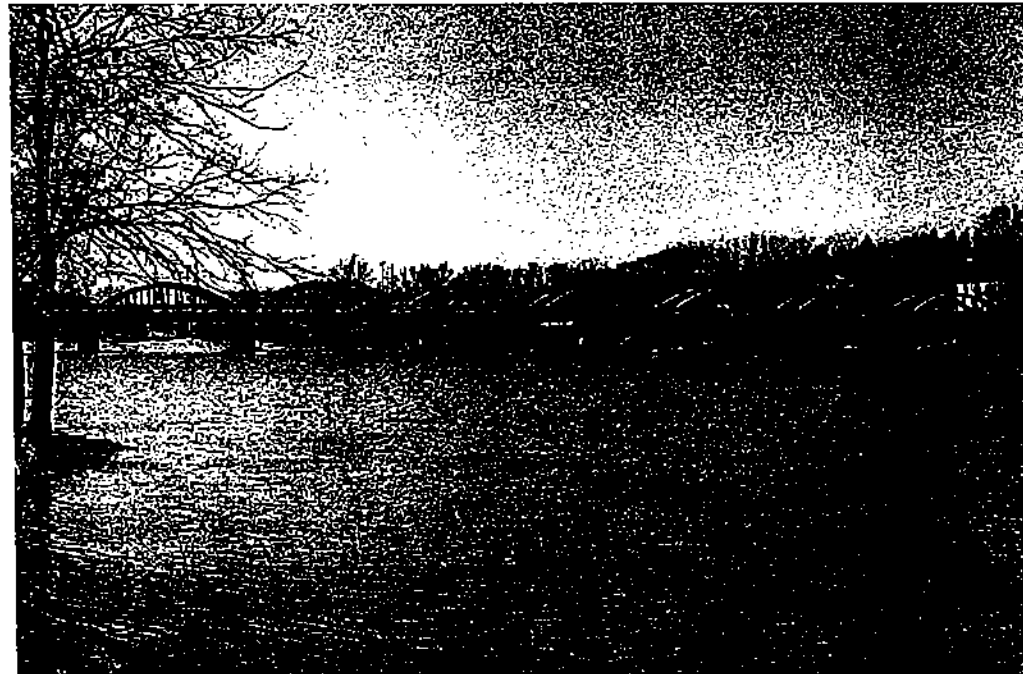
Plate 2. View of the Caledonia Bridge from the east
