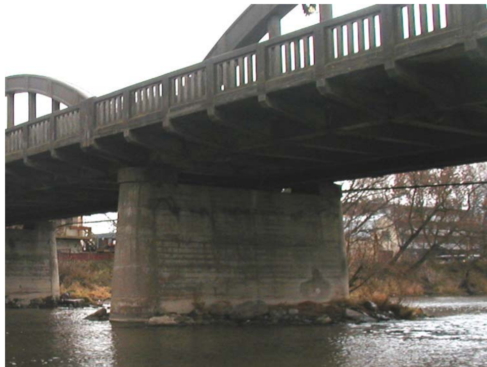
Pier No. 2, south face
