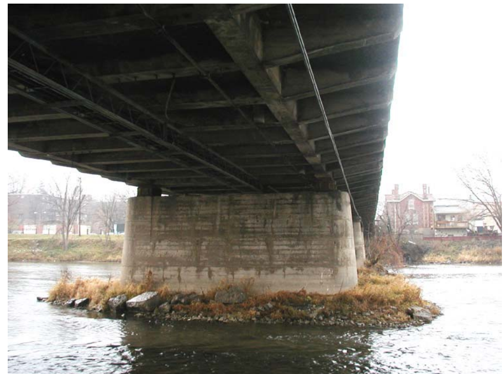
Pier No. 3, south face
