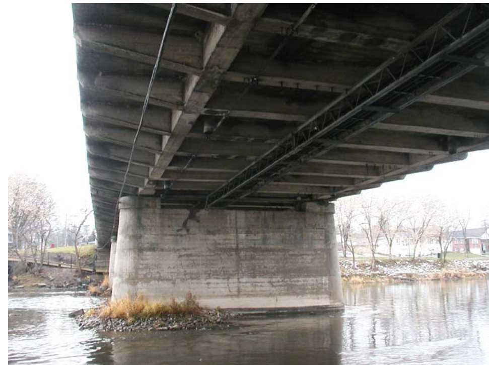
Pier No. 7, north face
