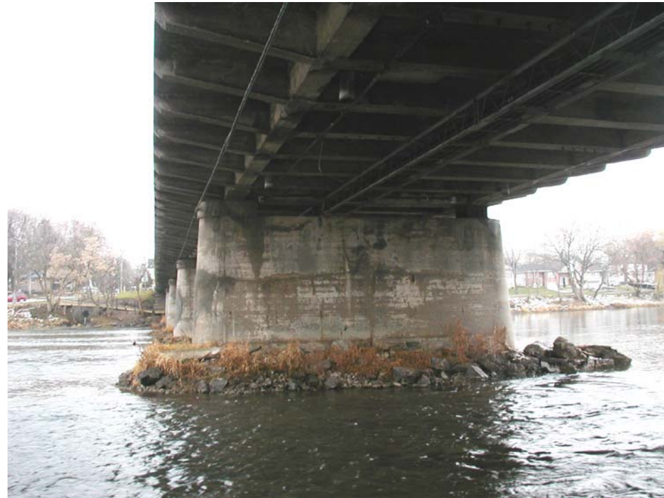
Pier No. 5, north face
