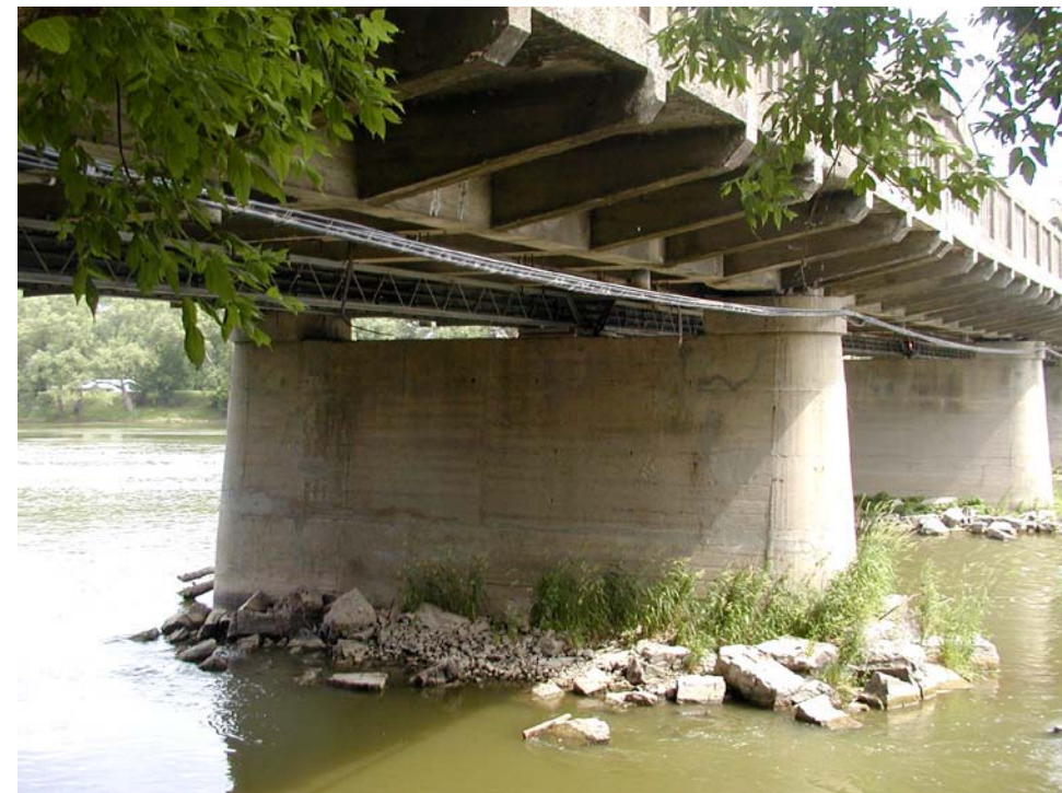
Pier No. 8, south face
