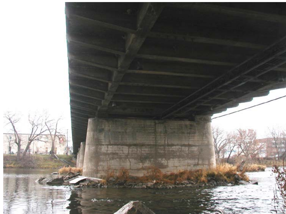
Pier No. 6, south face
