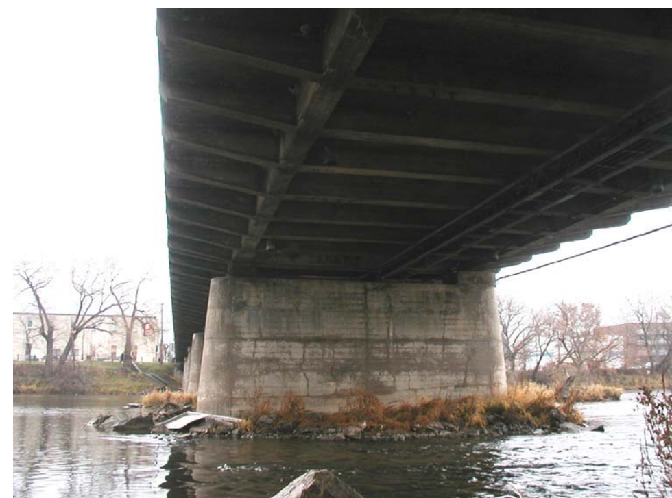
Pier No. 4, south face
